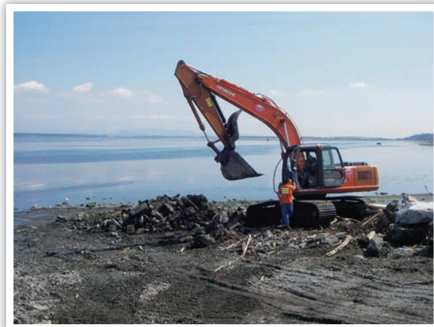
Removal of rock groin at March's Point
