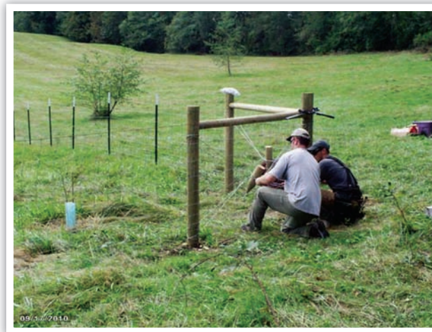
Fence being installed through CREP
