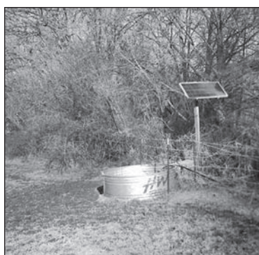
An example of one of the solar powered water pump systems.
