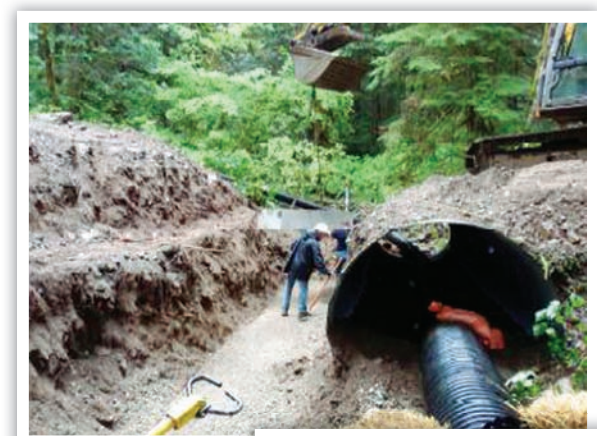
Culvert Replacement
