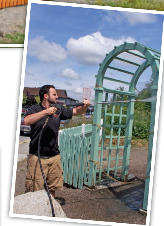
ABOVE - Brooks Carpenter of Rodda Paint pressure washed the garden fence and arbor in prep for a fresh new coat of paint.
