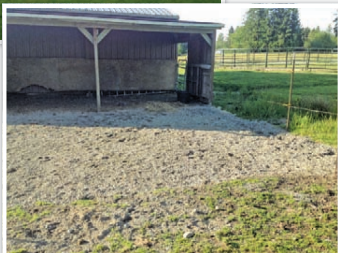
Confinement area after the implementation of a heavy use area protection project. Gravel in the confinement area reduces mud issues.
